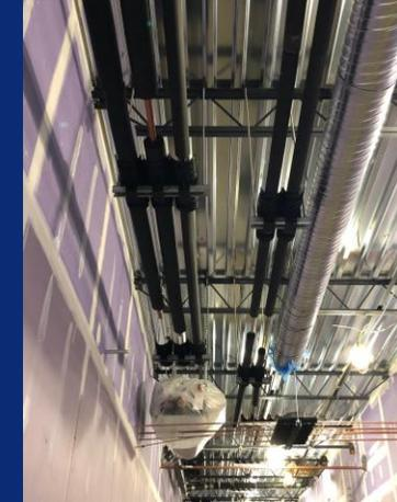
Line sets starting for 3<sup>rd</sup> level VRF system
