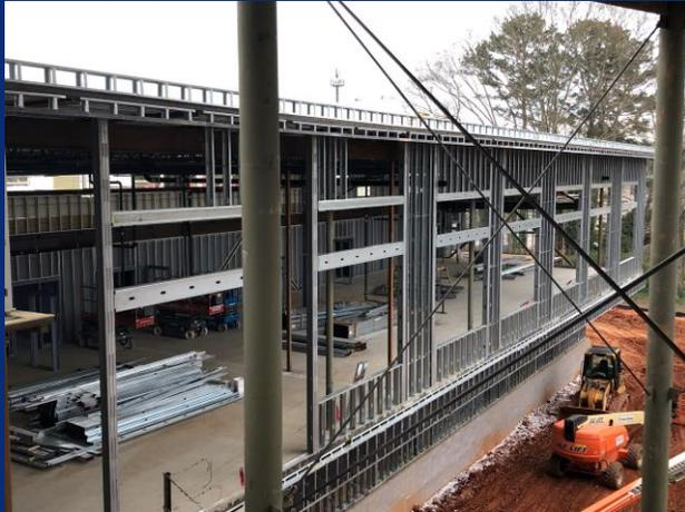
2<sup>nd</sup> level east exterior framing in progress
